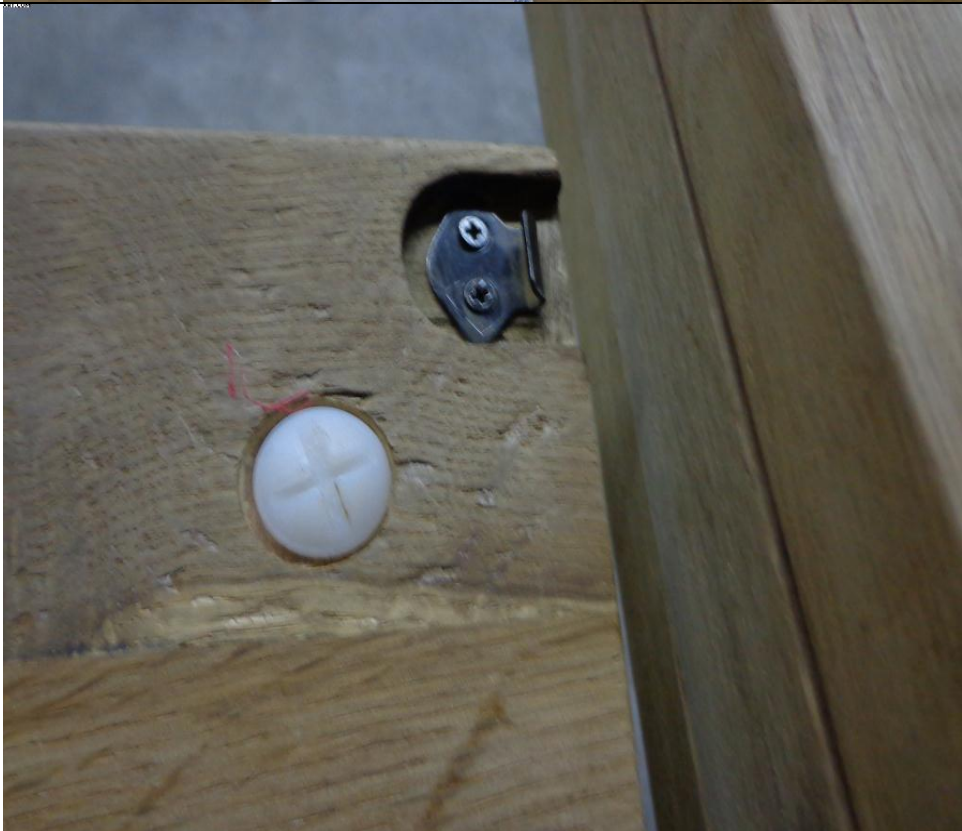
Catcher for lock of inlay. White bolt id to balance inlay compared to top.
