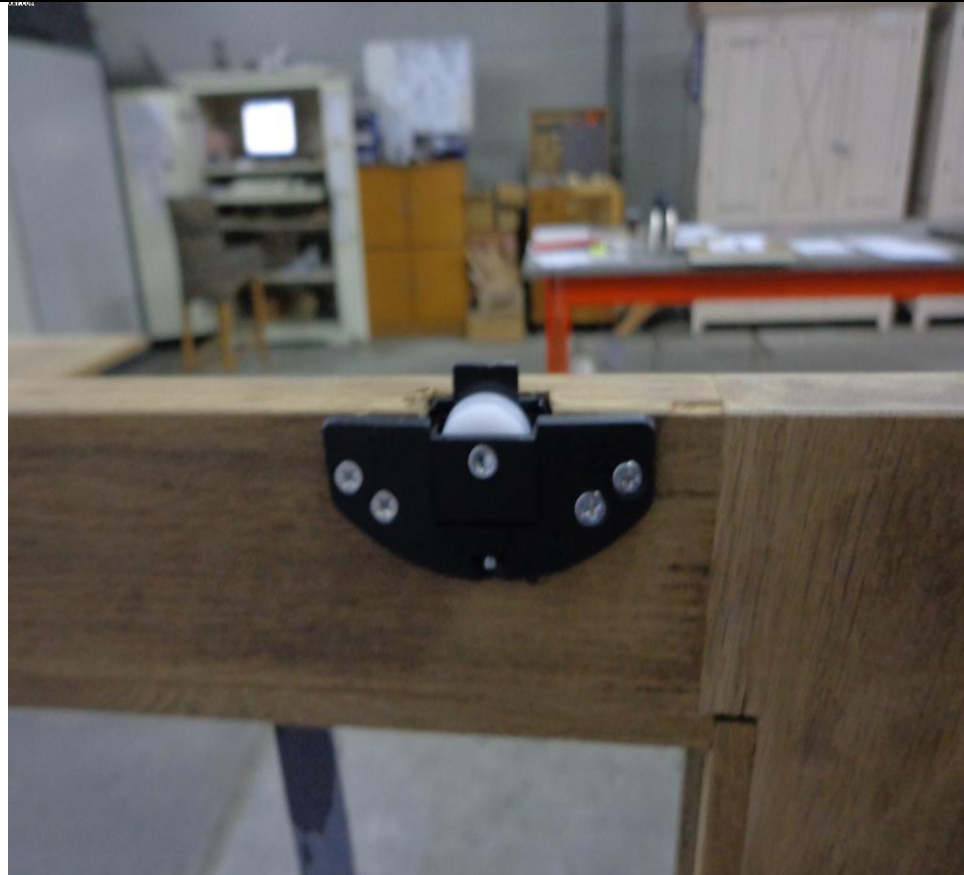
Wheel for easy sliding of sliding door.
