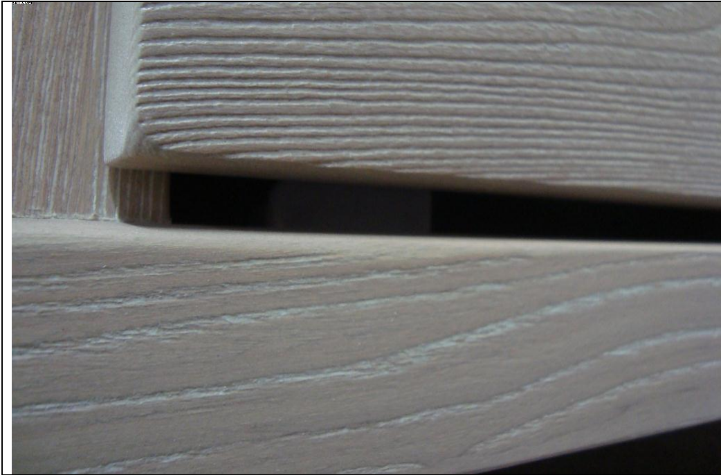
Space between doors and frame
