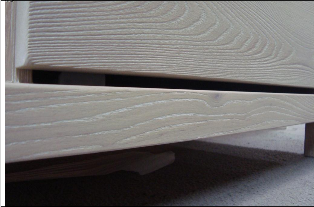
Space between doors and frame
