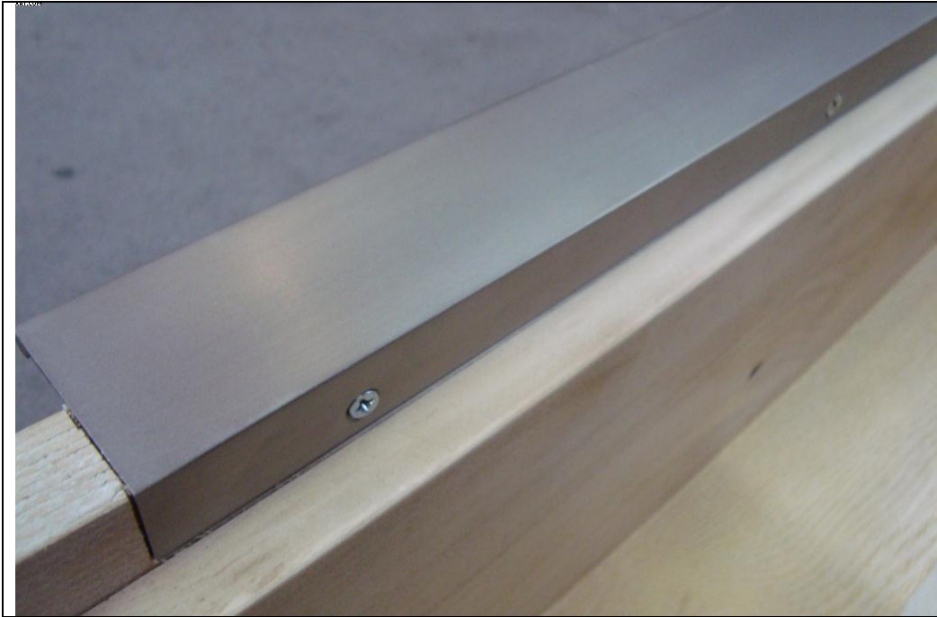
Screws for assembling the grip on the drawer
