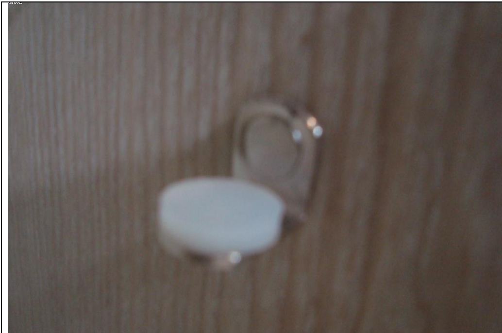
Metal pin with silicon to support glass-shelf
