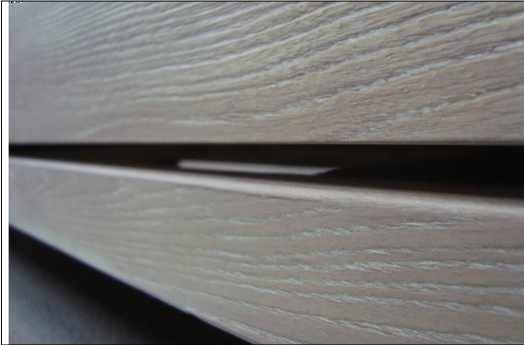
Space between doors and frame
