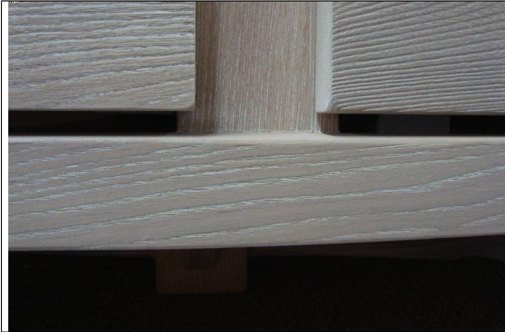
Space between doors and frame
